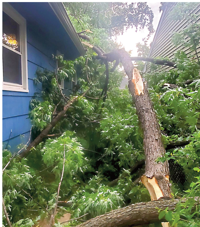
Use caution when approaching storm damaged trees. If there are downed wires, stay clear and dial 911.
